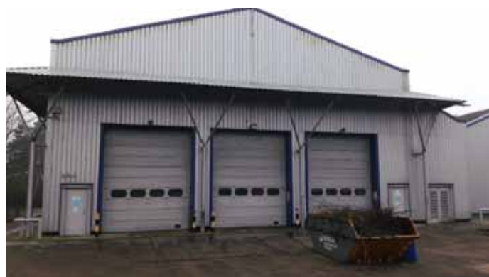
Three Bay Workshop (Crash Bays?)
