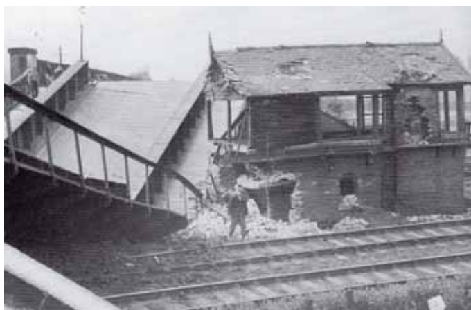
Two views of the Southcoates Lane railway bridge, destroyed by a bomb in July 1943 (Central Library Collection)
