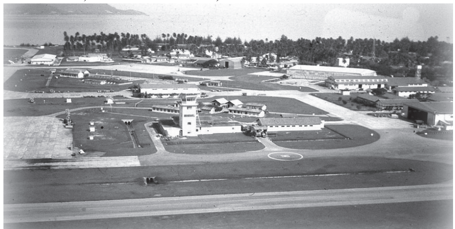
Aerial shot of Butterworth with ATC Tower and Crash Bay centre and Penang in the background
