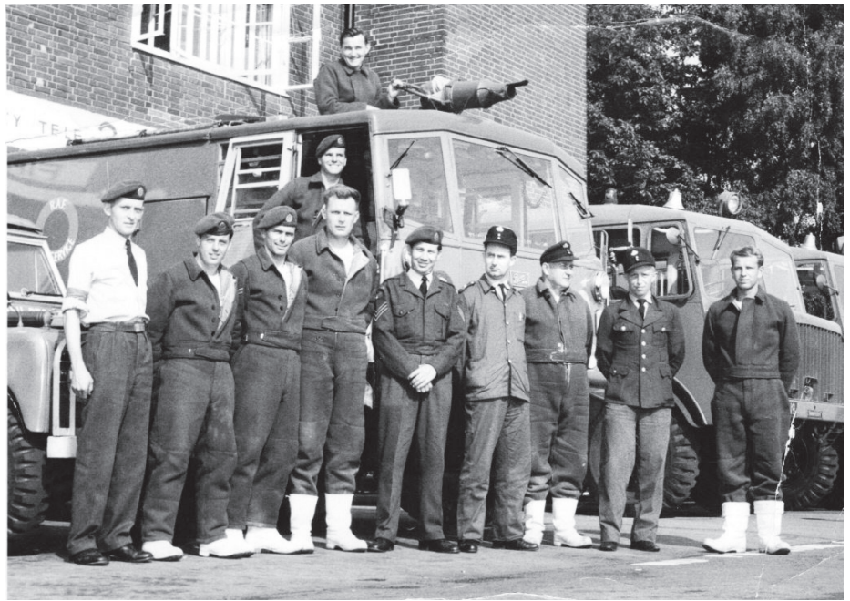
From left to right:- C pi. (in Control room), SAC Gallagher, Cpl Stevens (self), Paul German fireman, SAC Bernie Josling (in cab), German fireman (name unknown holding monitor), Sgt Dominic, Herr Phlanz, Fireman Willey Winkier, Herr Keller, Ferdi German fireman
