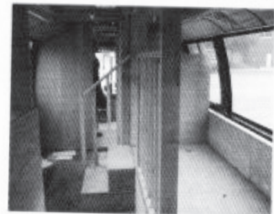
The two pictures above show the Interior conversion being carried out
