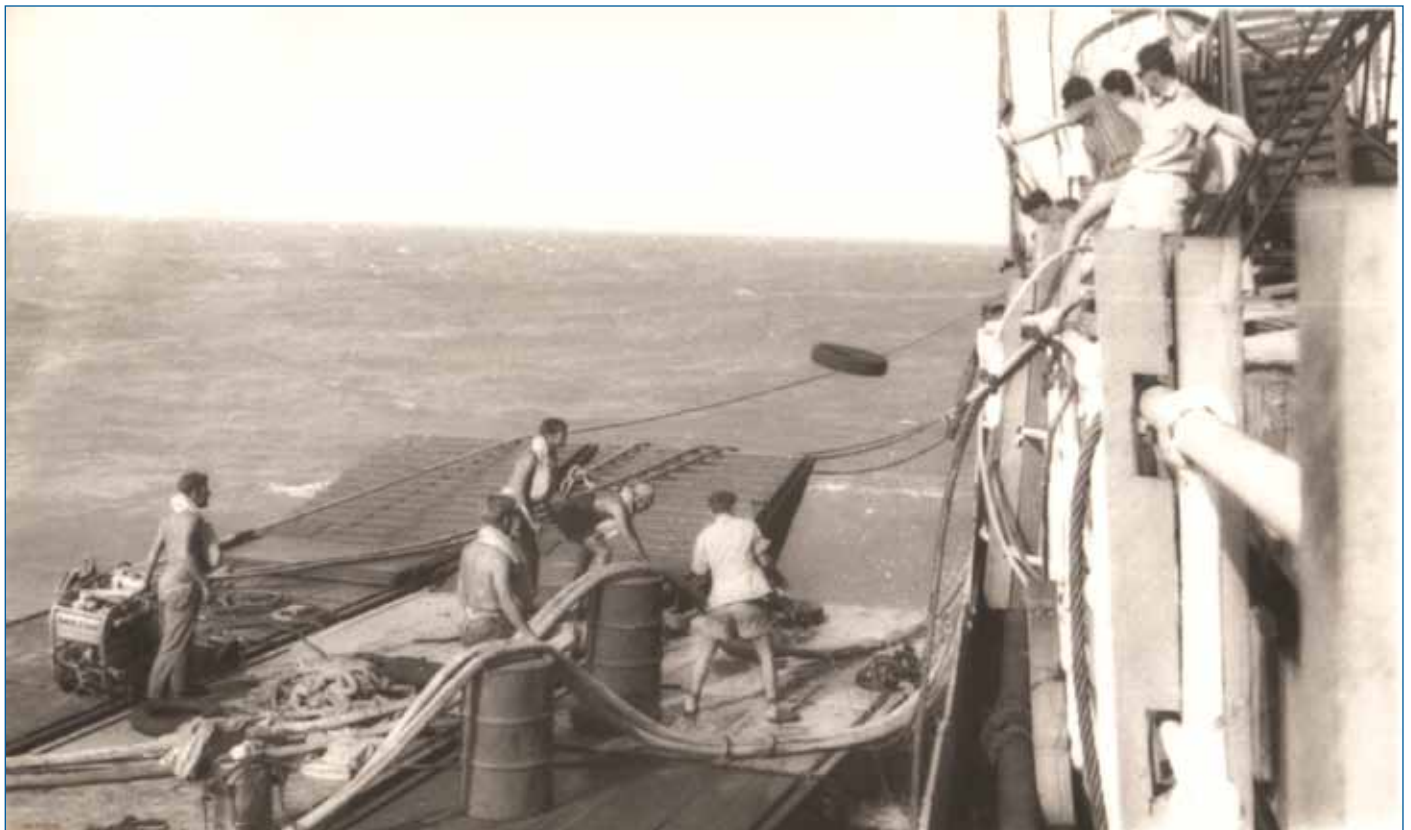
Rhino alongside Daphne, trailer pump detail getting water up to fire fighting detail Note missing front stardboard section
